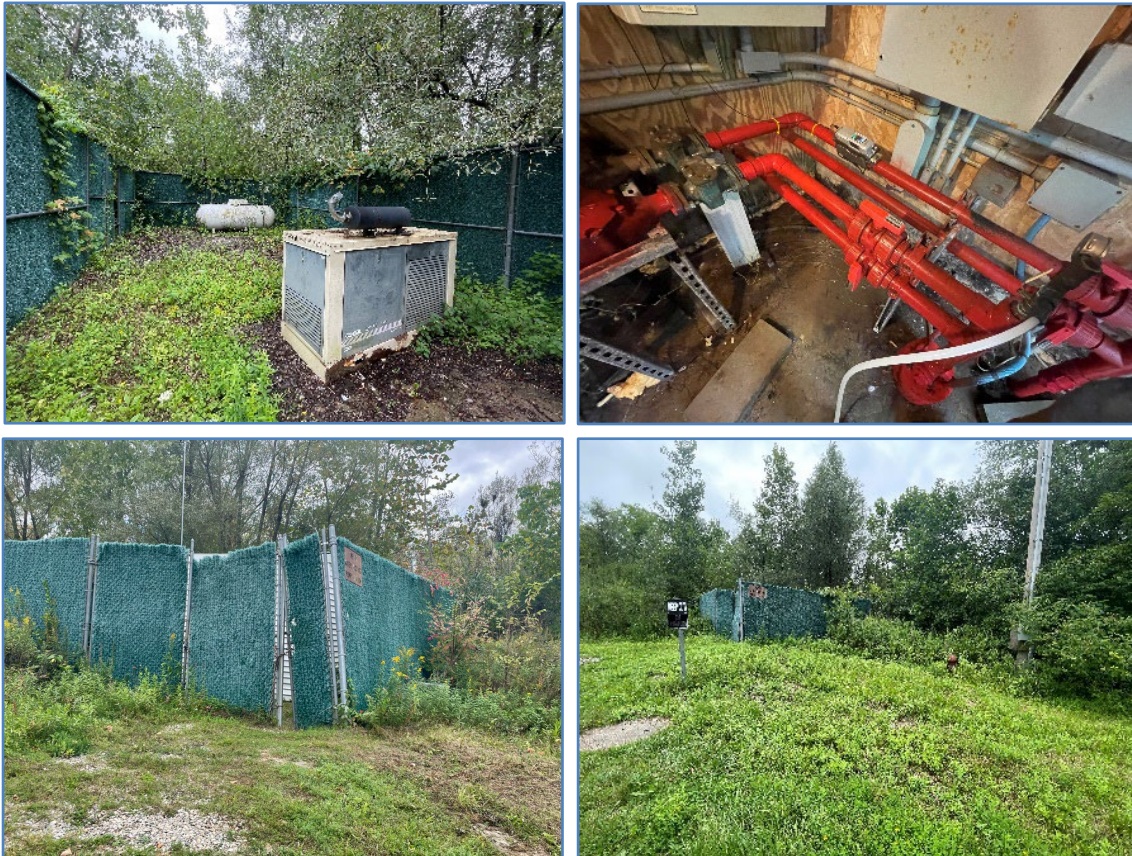
Figure 12. Lavelle Road Pump House and Fence Photos
