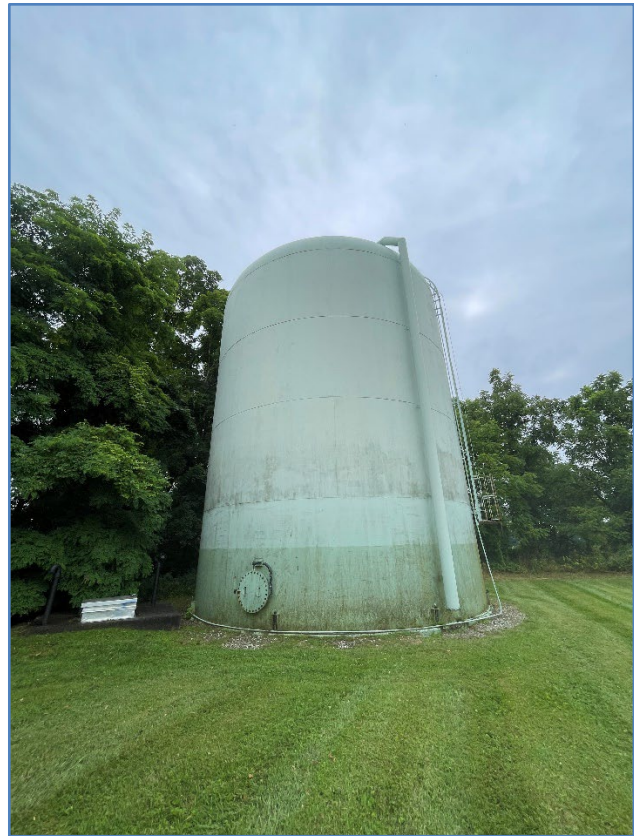
Figure 13. Photo of 200,000-Gallon Water Storage Tank
