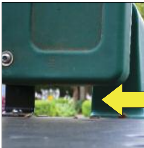
Examples of partially bound openings. Note, these examples are intended to illustrate the principle of partially bound openings and may or may not require testing.
