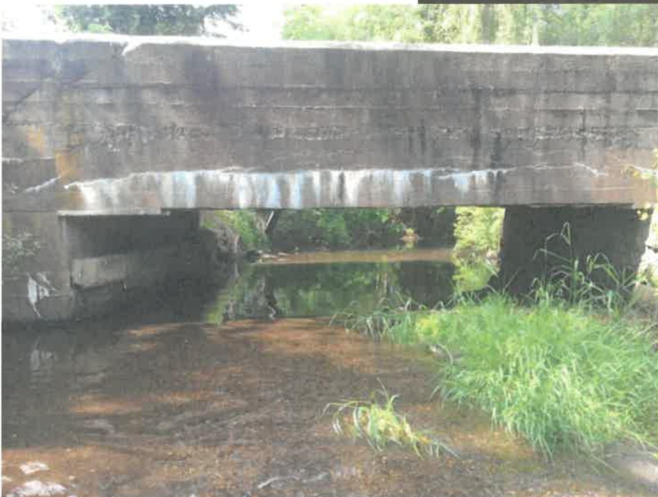
Right: Inlet of the current structure.
