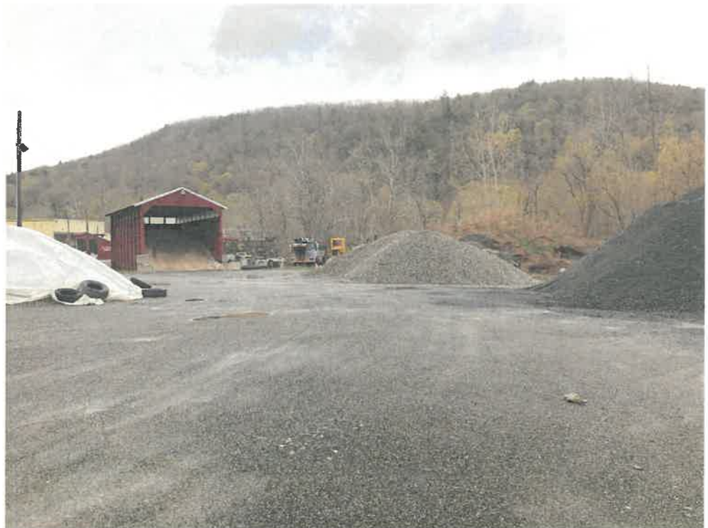
Right: Salt shed surrounded by large piles of sediment within floodplain
