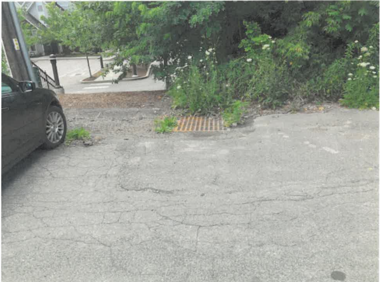
Below: Vegetated storm drain on opposite side of road
