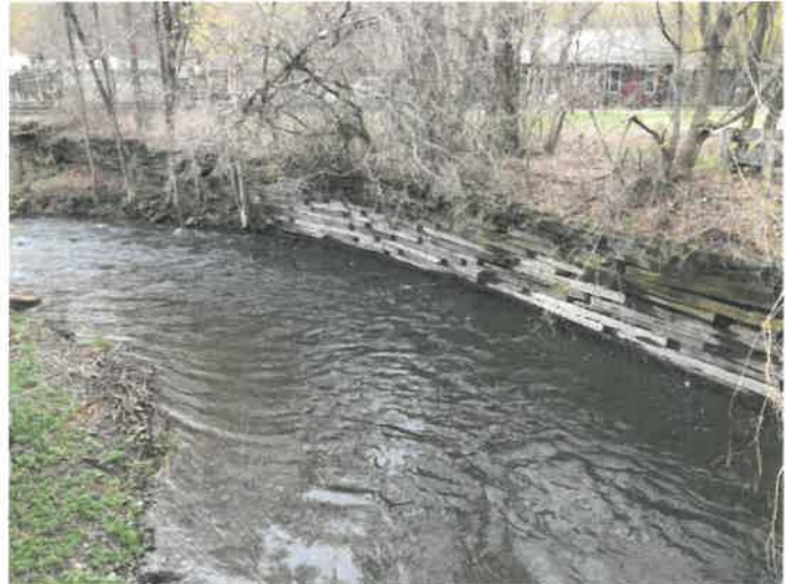
Retaining wall below parking area at Wassaic Park
