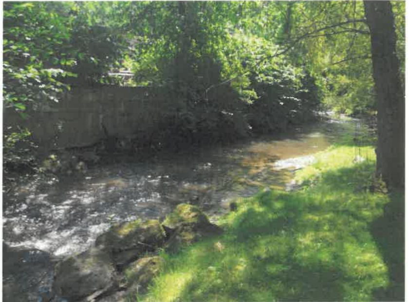
Fill in the Webatuck Creek floodplain behind retaining wall at North East Highway Garage, Village of Millerton.
