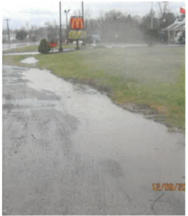
Photos (clockwise from top left): Stormwater accumulating in the parking lot and beginning to flow into Wells Brook; Stormwater flow heading for Wells Brook; Downstream end of stormwater flow entering Wells Brook; Stormwater on upstream side (CVS parking lot)
