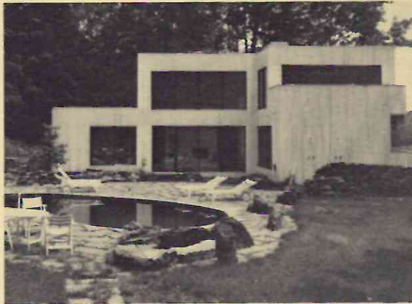
Behind the modern white house shown above, the black gunite pool, terraced gardens, and a private mountainview. Architect: Phillips Janson Group.
