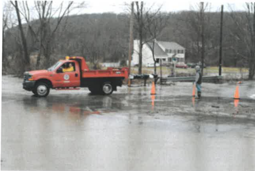
Cascade Brook overflowing Folan Road Bridge, April 16 th , 2007.
