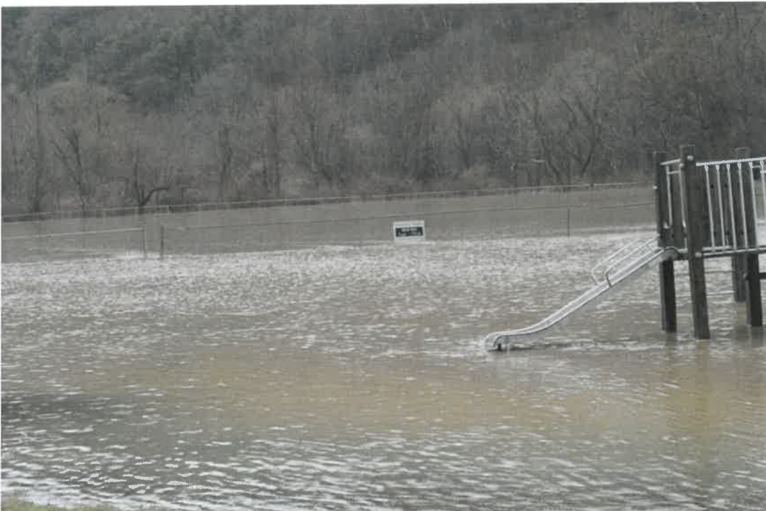
Wassaic Creek flooding the Wassaic playground April 16 th , 2007. Playgrounds, properly constructed, can be located on floodplains. Floodwater came over a 3' high berm.
